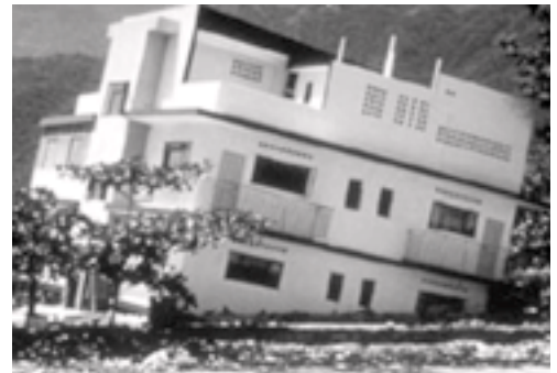
A partially sunken house illustrates the challenge of understanding how grains of soil interact with each other and under what conditions they will support structures. (National Geophysical Data Center)
