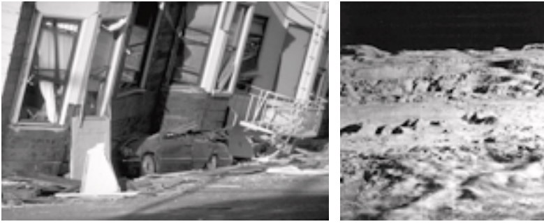
Figure 2. Partially sunken houses in San Francisco and the slumped sides of Copernicus crater on the Moon share one geologic fact: soil liquefaction. (USGS, NASA)
