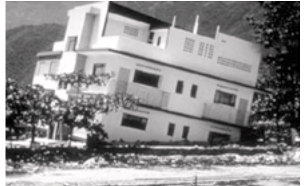
Figure 1. Excessive settlement in a building as a result of sand liquefaction. Earthquake of July 29, 1967, Caracas, Venezuela (National Geophysical Data Center)
